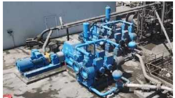
ABEL HMQ for cement paste, solid content > 75%
