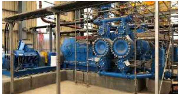
ABEL HMQ, thickened copper tailings at 77 bar
