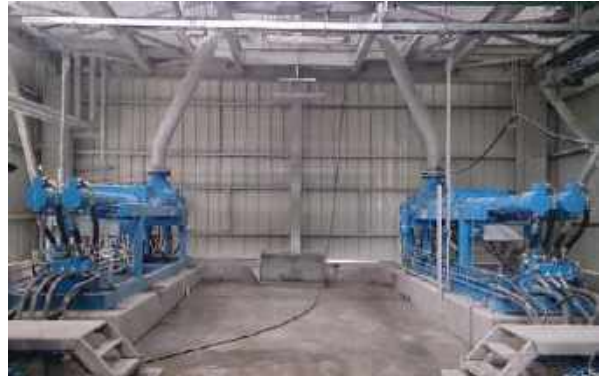
ABEL SH for mine backfilling at an altitude of 4800 m
