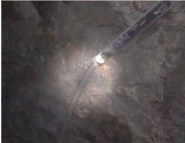
Paste discharge, continuous flow without pulsations
